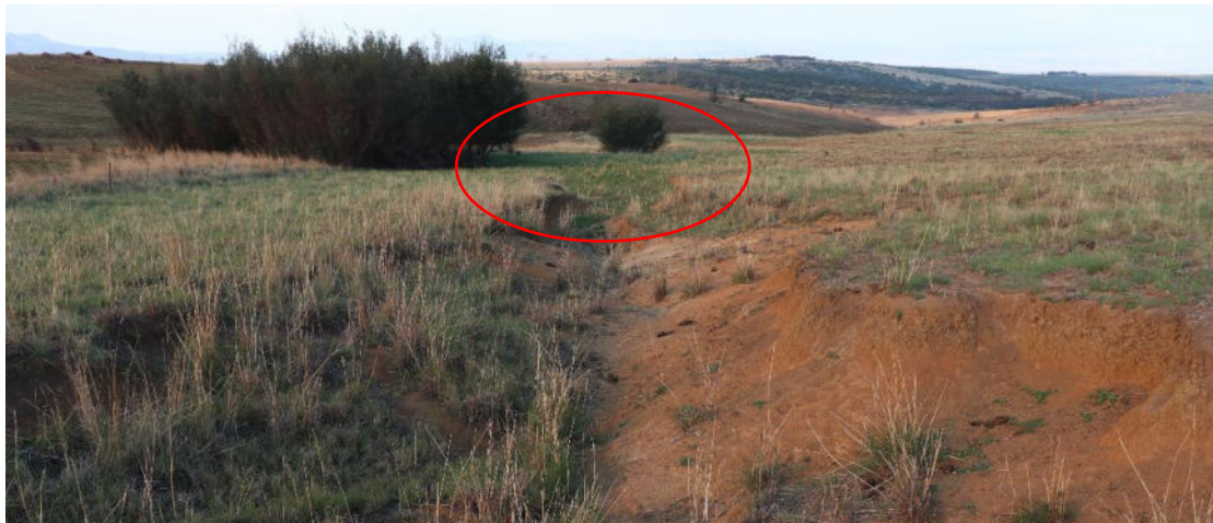
Figure 14: View of another seepage wetland (red), where head-cut erosion has progressed considerably and will eventually result in gulley formation. This is clearly resulting in significant impacts on the wetland.
