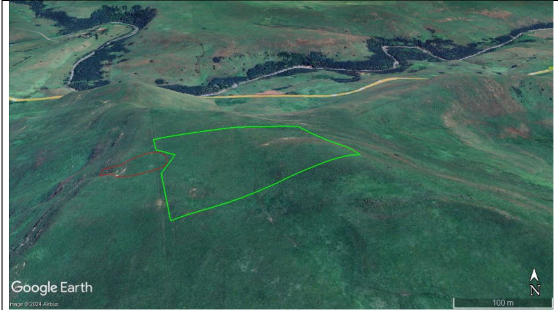
View of Site 4 with a small seepage wetland originating immediately to the east of the site. Impacts on it are therefore anticipated to be significant and a suitable buffer zone between the site and borrow pit would therefore have to be established.
